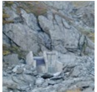
Intake in detail.
